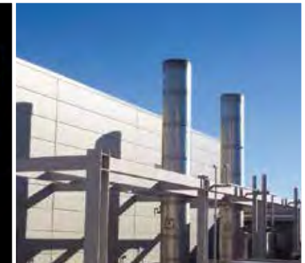
CPP offers exhaust/intake design testing
