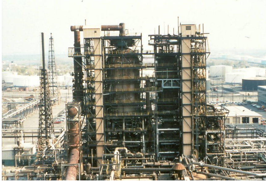
Figure 10. Typical lattice/porous type structure not treated by AERMOD/PRIME
